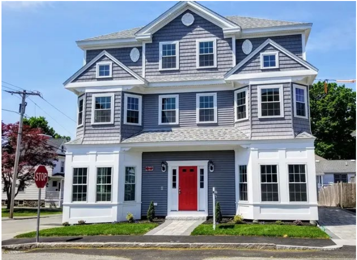
North Andover – Part new construction, part conversion into 6 ownership units
