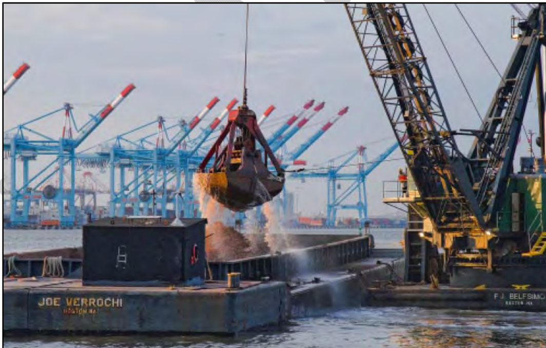
Figure 25 - Cashman Dredge F.J. Belesimo at work loading barge. 28 June 2019.
