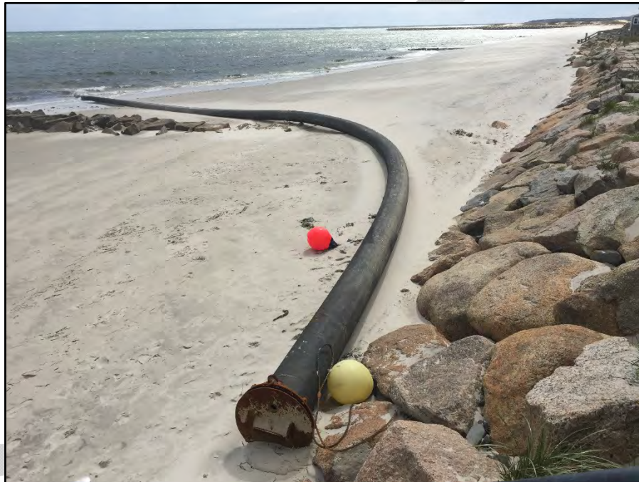
Figure 29. Length of HPDE discharge pipe coming ashore at local dewatering area, Yarmouth, MA, May, 2019.
