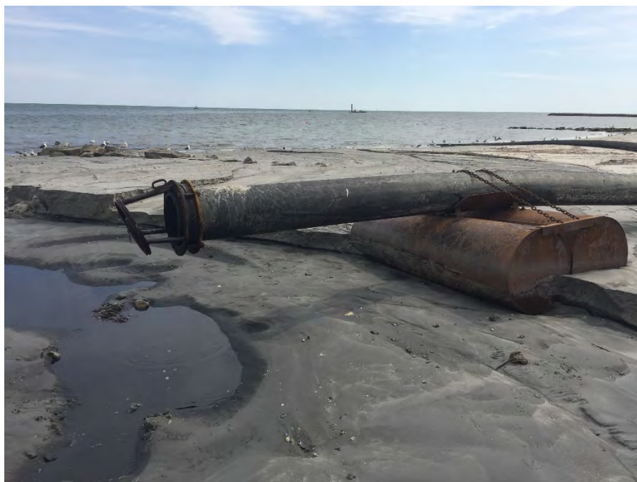
Figure 6 – Barnstable County Dredge discharge pipe – dredge superstructure visible in background, dredge pipeline sits on bottom of Nantucket Sound to minimize impacts to navigation.
