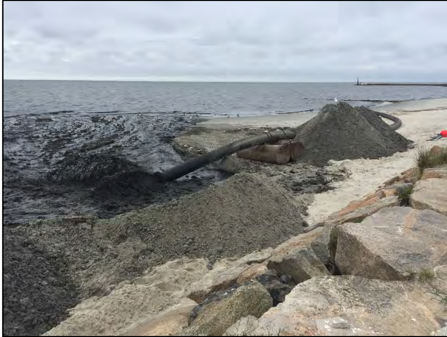
Figure 20 - Barnstable County Dredge Pipe discharges dredged material at dewatering site. Dewatered material is then stockpiled for beneficial reuse, May 2019.
