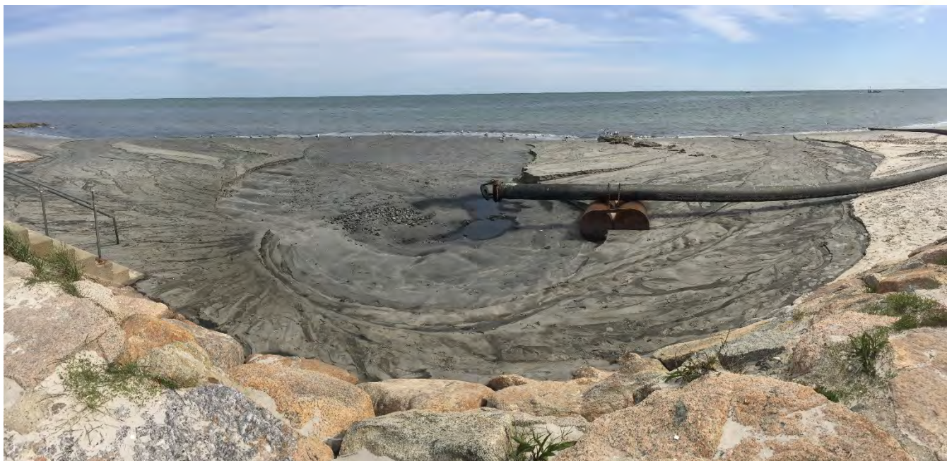
Figure 5 – Barnstable County Dredge dewatering site. As project continues, dredge spoils will accrete on beach.
