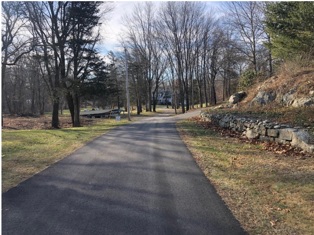
Looking up existing common driveway
