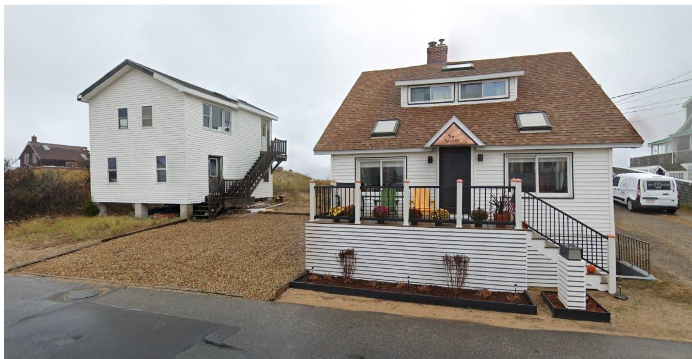
Primary frontal dune with newly installed parking area in front of 3 33rd Street. Vegetation removed from structure and parking area established at 108 Northern Boulevard. 2019
