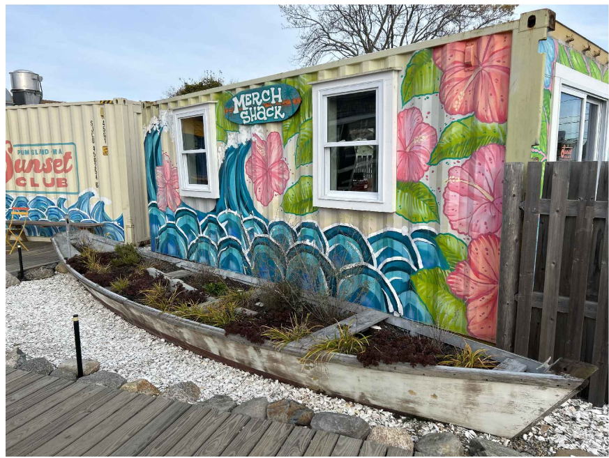
EXISTING ( UNPERMITTED ) MOBILE CONTAINER ACTUAL PHOTOGRAPH SCALE: N.T.S.
