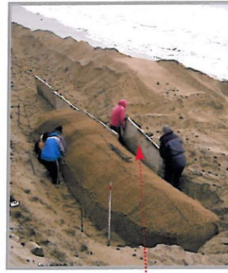
Forms are moved into position to start another tube, and sand is back filled behind the tube.
