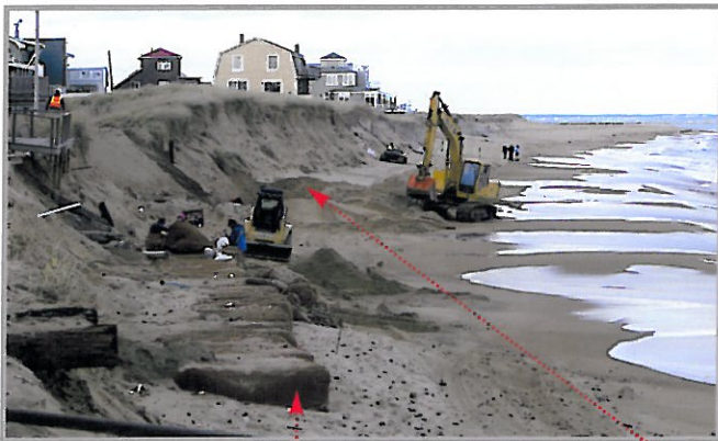
A second team has started constructing layer 1 tubes in a southerly direction; and layer 2 is being added in the foreground.
