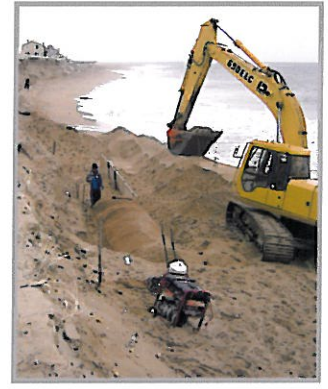
Forms are moved into position to start another tube, and sand is back filled behind the tube.
