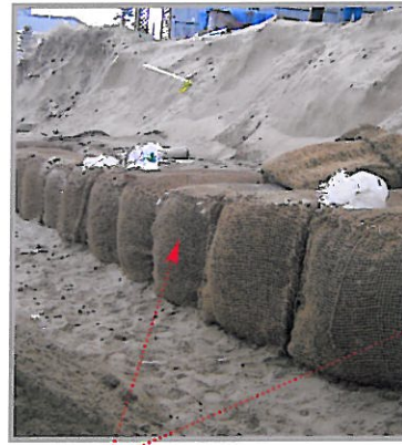
The 2 nd layer consists of 6 foot long tubes constructed "in place" at a right angle to and on top of the layer 1 (base tubes).
