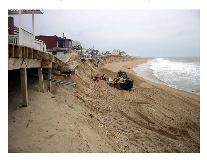
The erosion of beach and dune that has been occurring immediately north of the center parking lot groin now directly threatens public infrastructure as well as private property. The current effort to reinforce the area consists of the placement of a "soft" biogradeable structure to buttress the remaining dune. While It does not solve the erosion problem, it should greatly reduce the loss of sand from the dune during storms.
