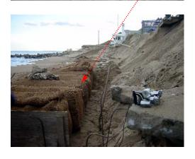
December 5, 2008 Installation of the second layer of 6' tubes has been completed to the northern terminis and is being extended southward to the groin.
