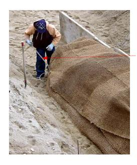
On the left the installer is seen stitching the end closed. Note the length of coir twine in his right hand.
