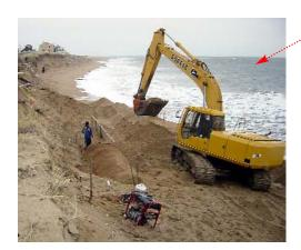
To the left the tube is being back filled with sand until it is completely covered. It abuts a tube on the near end that was placed earlier and will in turn abut the tube that will be placed where the forms are set at the far end. Eventually a second parallel line of tubes will be placed and these will form the base of the structure.
