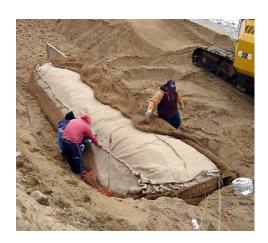
When the burlap has been stitched, the coir mats are pulled over and hand stitched together using long curved "needles" and coir twine of the same diameter as the warp and weft of the mat.
