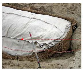
Once the sand has been added the burlap flap that had been draped over the form is folded over the sand and the shoreward edge of the burlap are pulled together and folded to form a seam. A portable electric sewing machine is used to stich the seam closed, and then to close the ends. This image shows one end of the tube after it has been closed.
