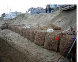
December 2, 2008, several additional tubes have been placed and a second team has started to the north constructing bags in a southerly direction. The second layer of tubes have been placed. These are 6 foot long and have been placed at a right angle to and on top of the tubes shown in the proceeding pictures.
