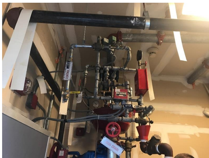
Figure 26: Main Service Entrance Sprinkler Room Fire Alarm Devices
