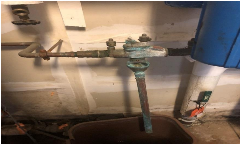
Figure 2: Reduced pressure backflow preventer for the HVAC boiler make-up water
