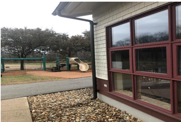
Figure 3: Typical exterior roof gutter and downspout
