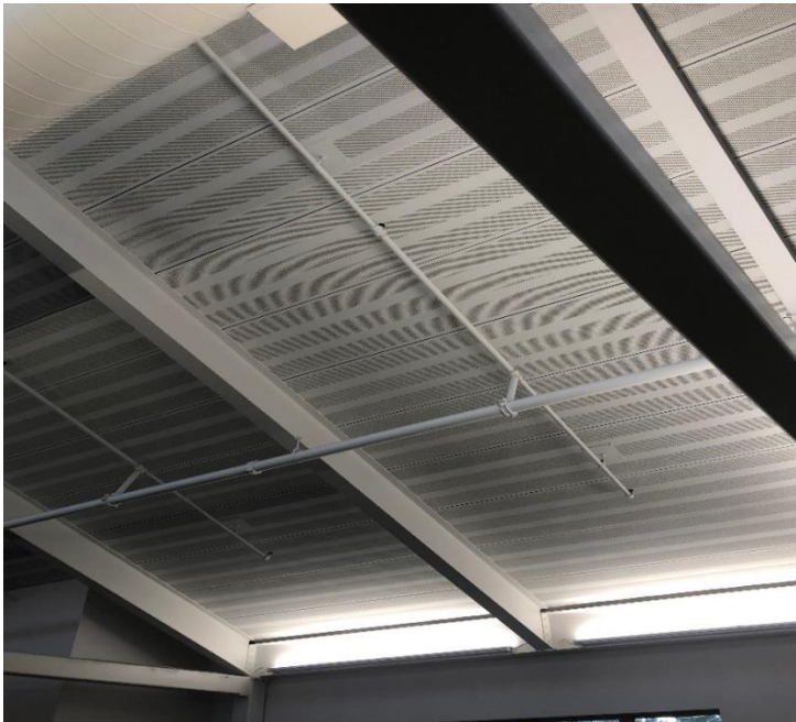
Figure 7: Typical exposed and painted sprinkler piping
