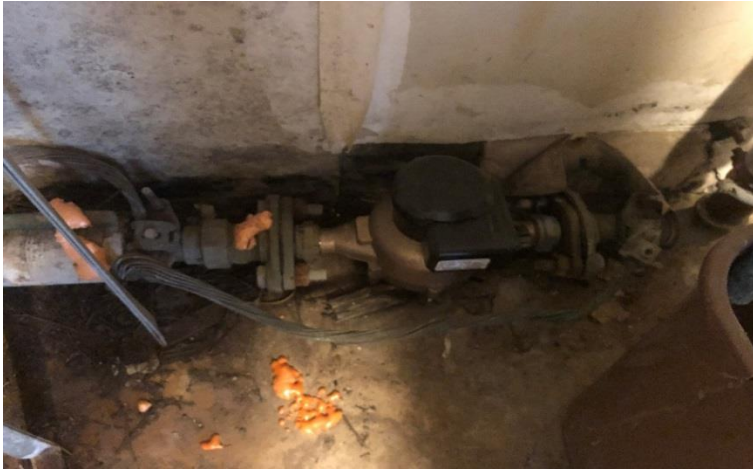
Figure 1: Domestic water meter within the sprinkler room
