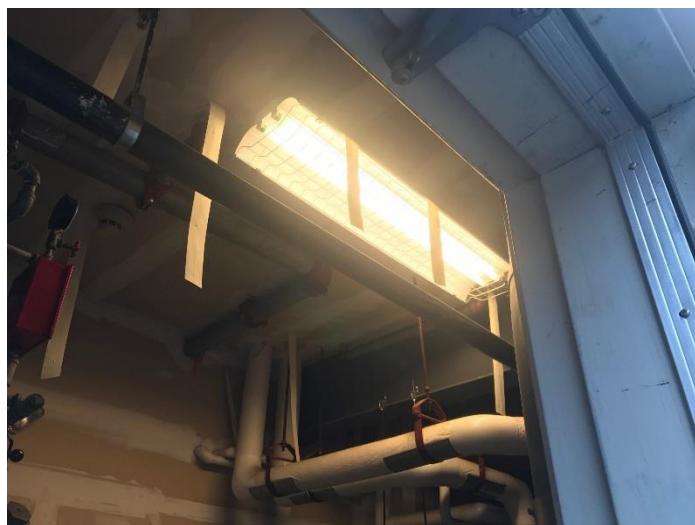
Figure 10: T-8 Fluorescent Industrial Fixture-Sprinkler Room
